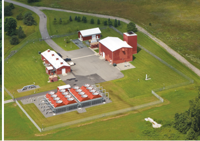
Dover, NY Compressor Station
