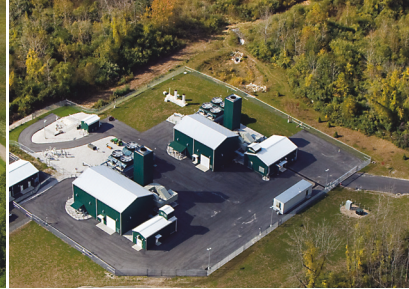
Brookfield, CT Compressor Station
