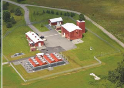
Dover, NY Compressor Station
