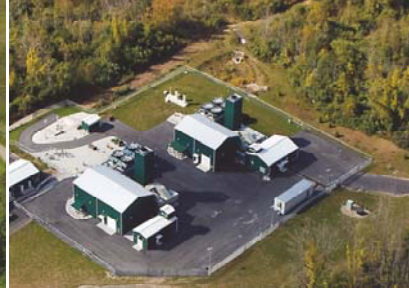
Brookfield, CT Compressor Station
