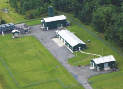
Athens, NY Compressor Station
