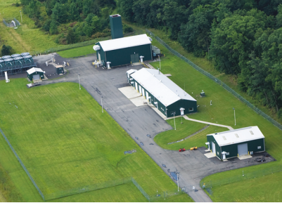
Athens, NY Compressor Station
